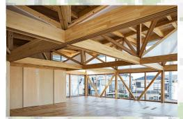
Reference of a floor plan that have flexible function using walls that are movable for different use. the whole house even the stairs and the elevators shafts are made of wood, so its easier to take the construction down one day.
